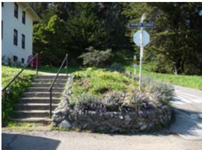
Stone retaining wall
