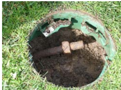
Subsurface threaded metal rod with bolt (possible remnant of former Alameda arch) (D.42)
