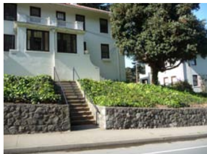
Stone retaining wall (A.38)
