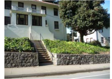
Stone retaining wall (A.38)
