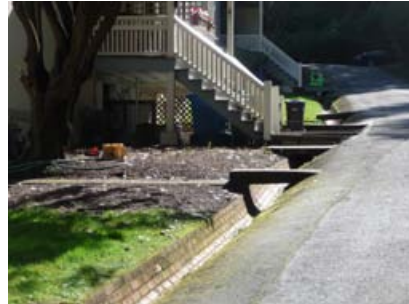
Brick drainage gutter (A.35)
