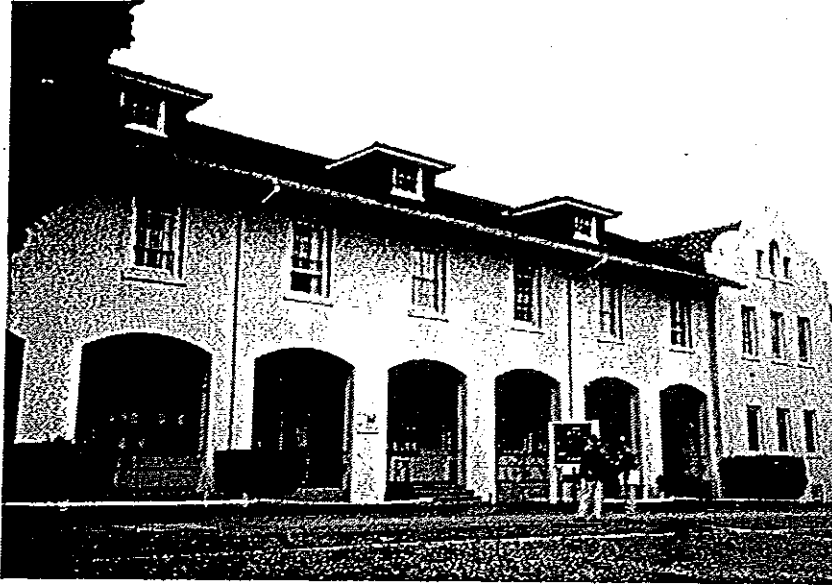
View from the Southeast
